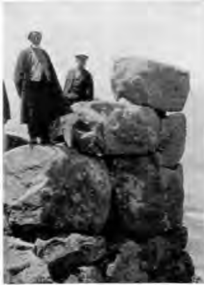
FIG. 142.—Aghaya Kaleh. Detail of the wall
