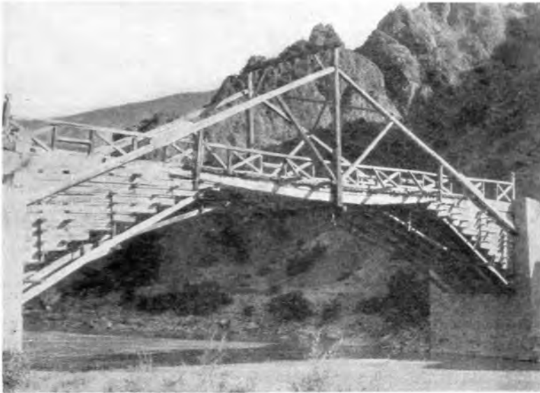
FIG. 153.—Bridge over the Kelkid Irmak
