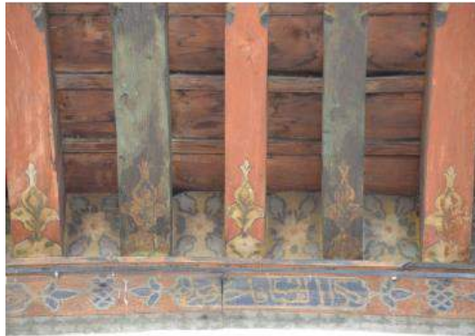
Figure 5 : Wooden ceiling with Painting decoration
